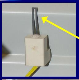
Remove and discard the old ignitor. Insert the new ignitor into place being sure to not touch the wire filaments.
