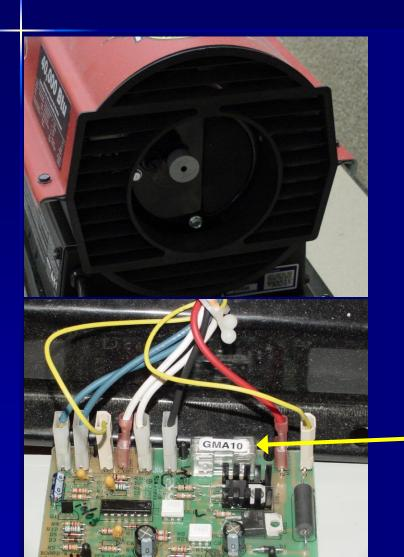
Replace the end-cover guard, slide the uppershell back on, and fasten in place. Test fire and look through the end cover towards the ignitor. You should see a glow if the ignitor is good. If the ignitor does not glow, check the fuse on the control board. Replace if necessary.
